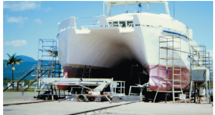
A typical slipway operation painting a luxury twin hull vessel using BlastOne equipment.
