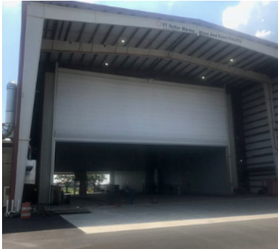
THE FRONT OF THE NEW BLAST AND PAINT FACILITY
