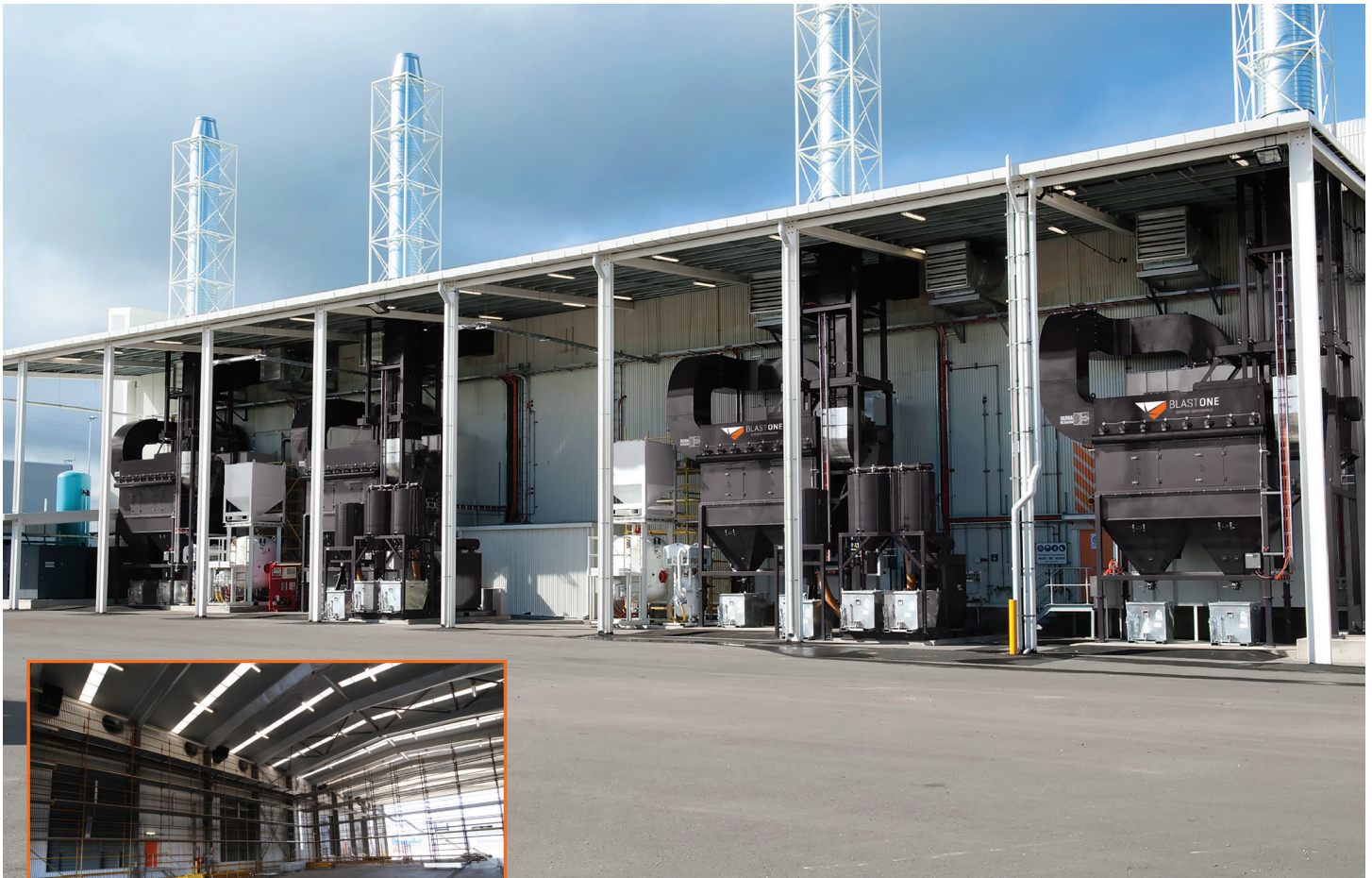
A TYPICAL LARGE BLAST AND PAINT HALL FOR SHIP SECTIONS: 75 FEET WIDE X 45 FEET HIGH X 180 FEET LONG
